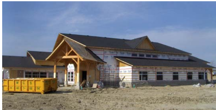
Spring has finally arrived in Ontario! Exterior work can begin soon.
